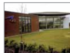
ECTS building in Burgess Hill, UK
