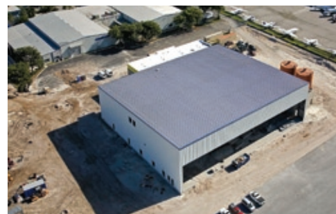
Service Center - Ft. Lauderdale - Hollywood International Airport, Ft. Lauderdale, Fla.
